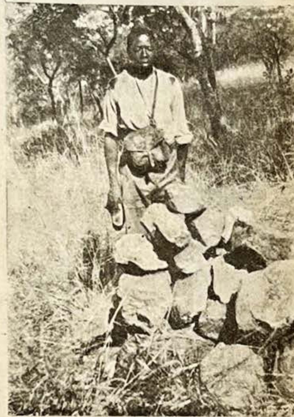
Erecting a Beacon for the New Mission Site at Belingive.
