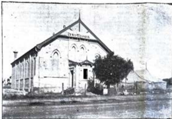
NEW CHAPEL AT PROSPECT, SOUTH AUSTRALIA.
