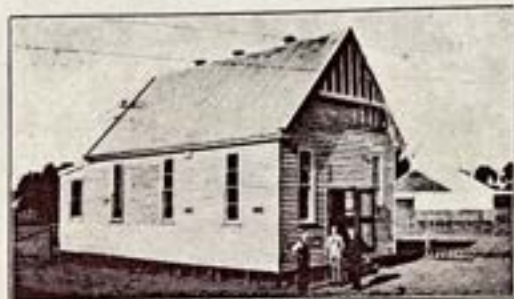
Recently-erected Building at Rochester, Vic.
