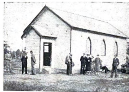
The Highcroft-Tunnel Bay Chapel.
