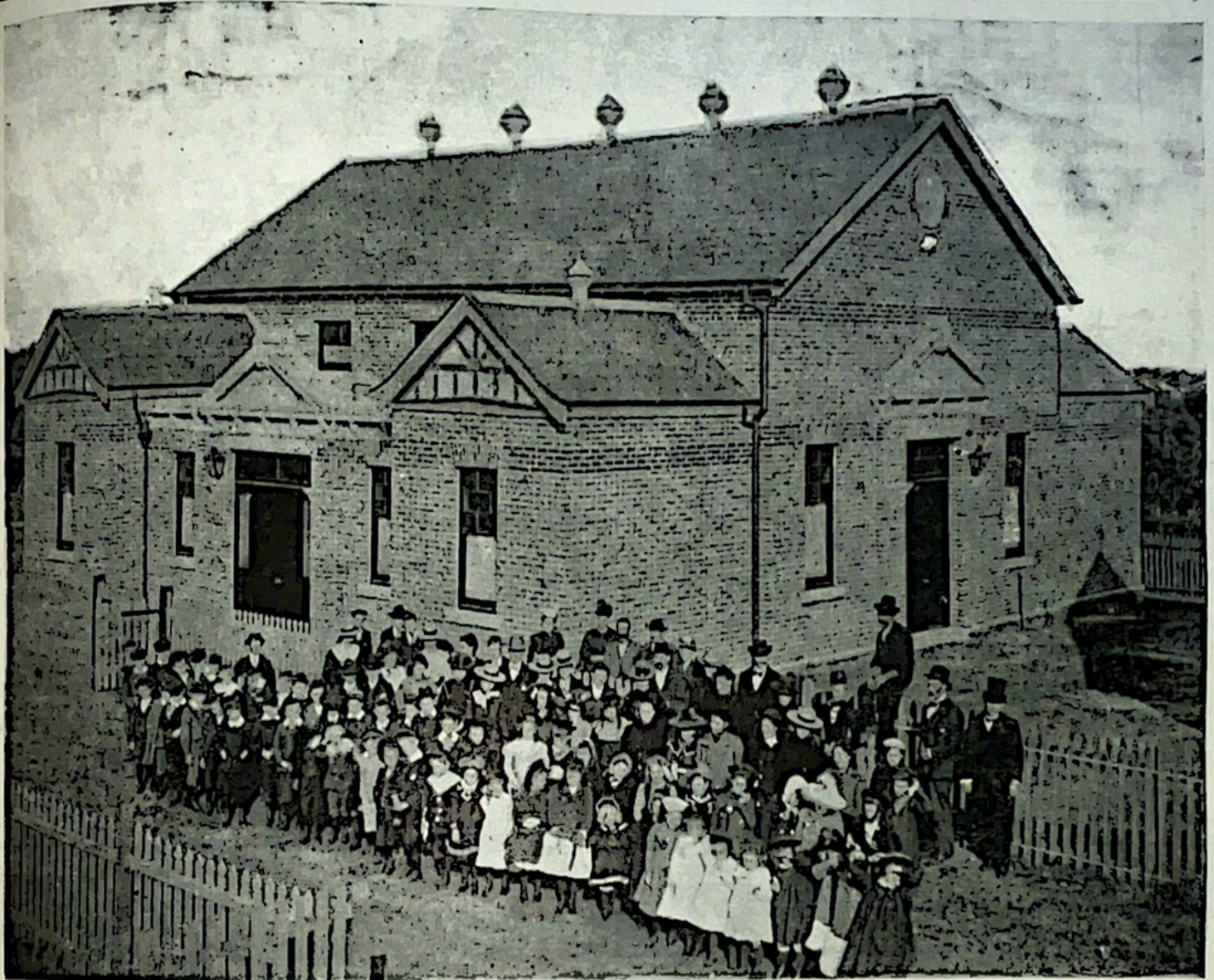
NEW LORD'S DAY SCHOOL BUILDING, CHELTENHAM.
