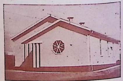
Building at Morwell to-day.
