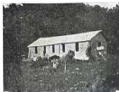
The New Chapel, Almost completed, Banmatmat, Sth. Seas.
