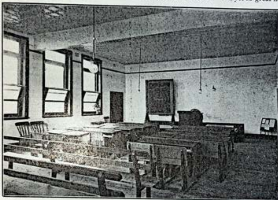
A Class Room in the New Building.
