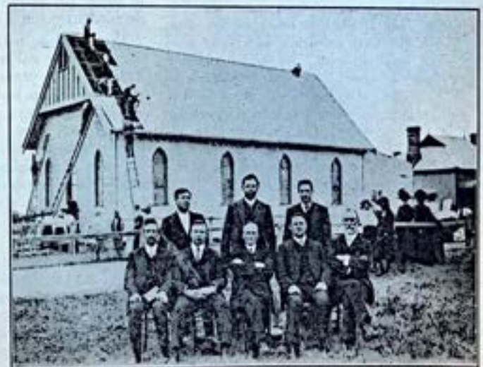
Finishing Roof.—5.30 p.m.
