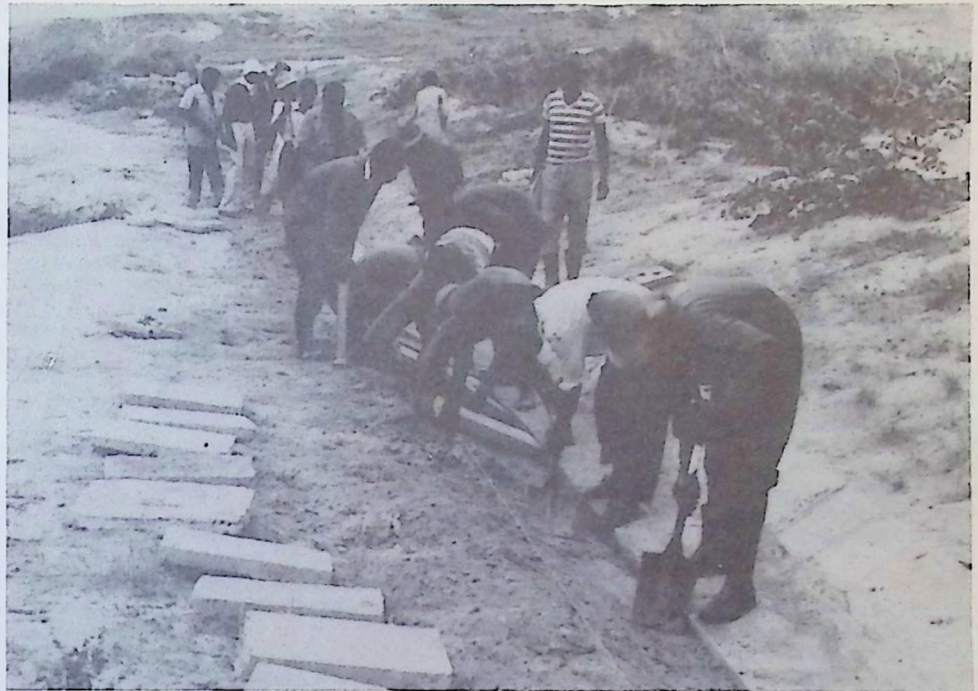
Villagers in Garlya, Bulawayo Diocese, working together to build an irrigation canal
