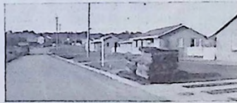
First Houses to be occupied in Yarralumla Creek Valley.
