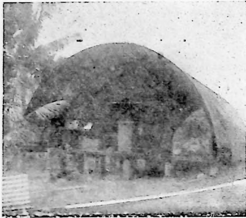
Mr. and Mrs. Smith's home before completion, Ranmaicat, Pentecost, New Hebrides. This is a converted army hut, dismantled on Santo and shipped to Pentecost. Mr. and Mrs. Smith now live in this building.
