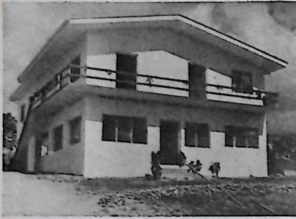
VILA CHRISTIAN CENTRE Fellowship Hall, lower level. Pastor's house and transit quarters upstairs.
