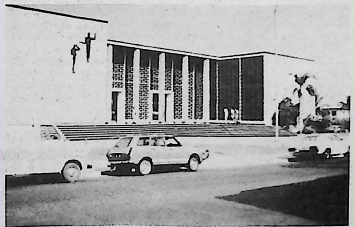
The Law Courts, part of Darwin's fine rebuilding programme. — "A.C." photos.
