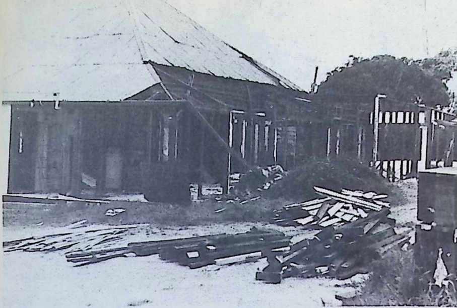
Building being demolished for Armadale-Kelmscott church.
