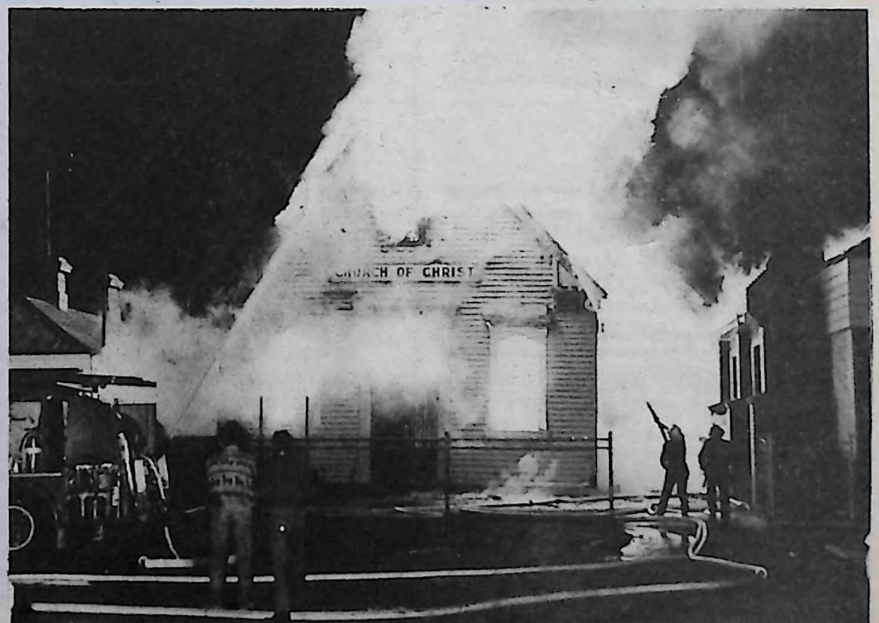
Ian Corlett (minister) and Barry Hamond (Secretary) watching firemen fighting the blaze just before the roof collapsed.
