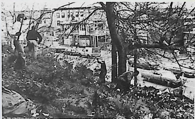
Clearing site for Housing Co-operative
