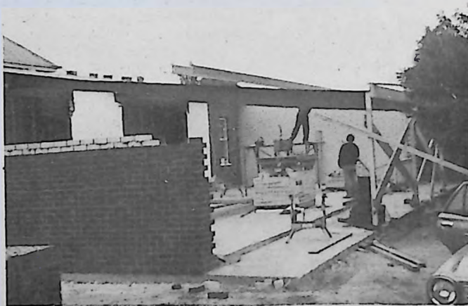
Bricklayers at work on the hall extensions at Maylands church.
