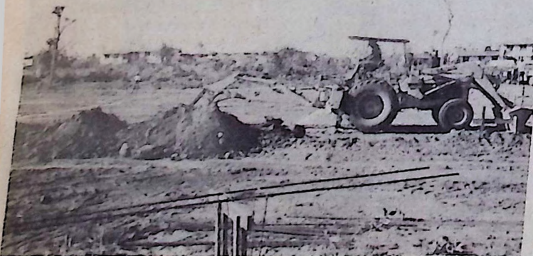
Digging the foundations
