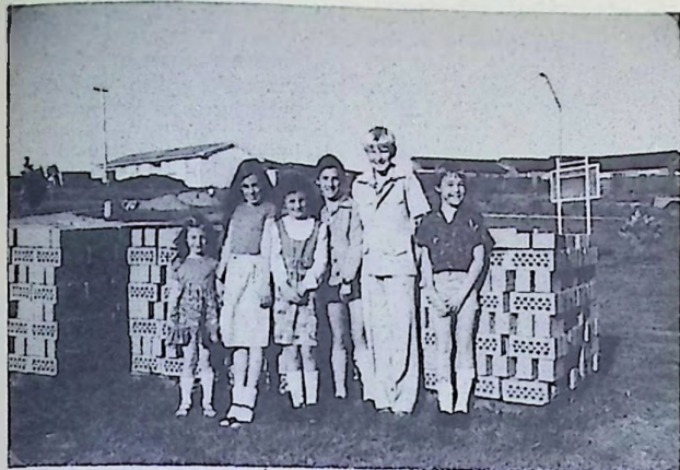
Building blocks of the Orange Church.
