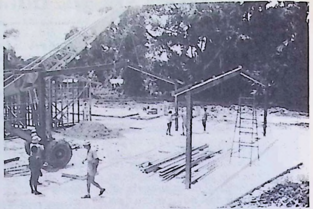
Steel frames go up
