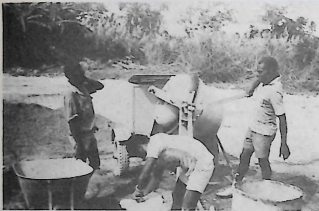
Mixing concrete
