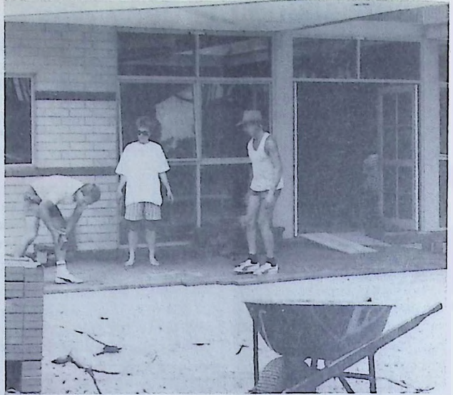
Members working on the paving
