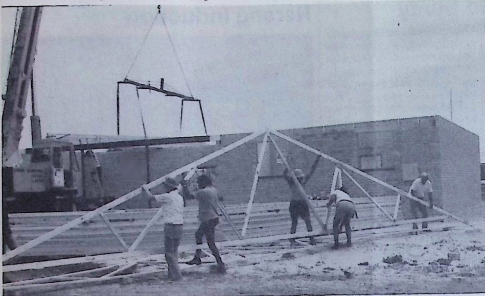
The first roof truss goes into place
