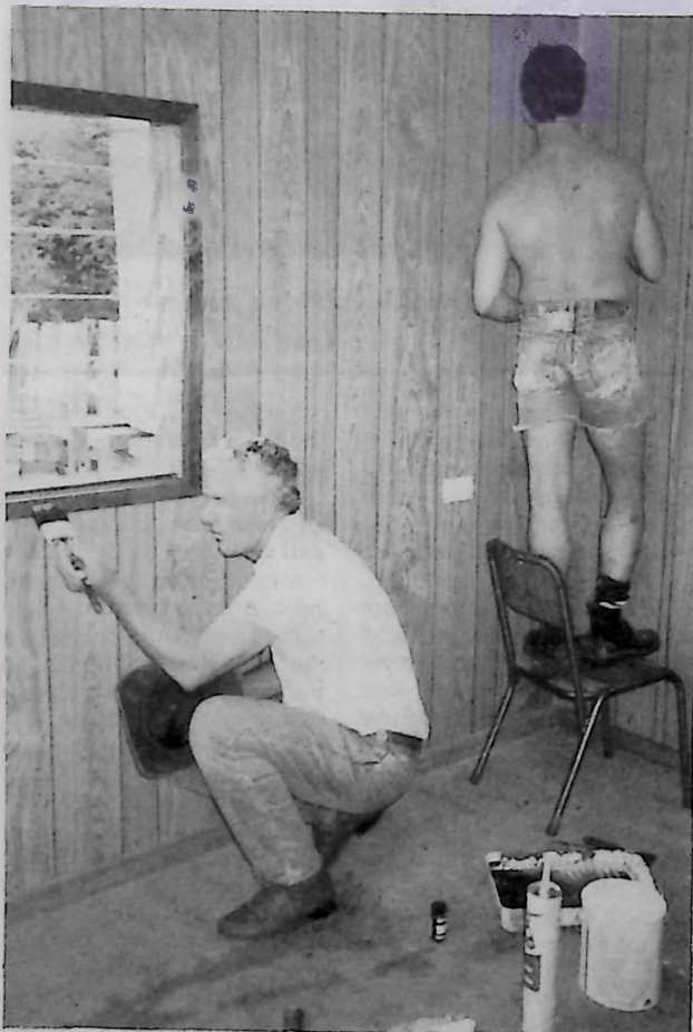
Finishing touches to new office, once an unlined garage
