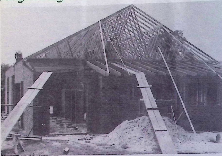
New building at Blaxland under construction
