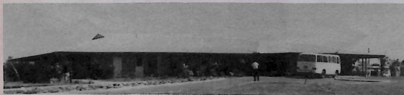
Frail Aged Hostel, Carnarvon, WA
