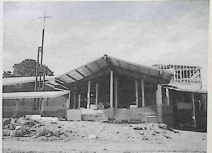
New worship centre under construction
